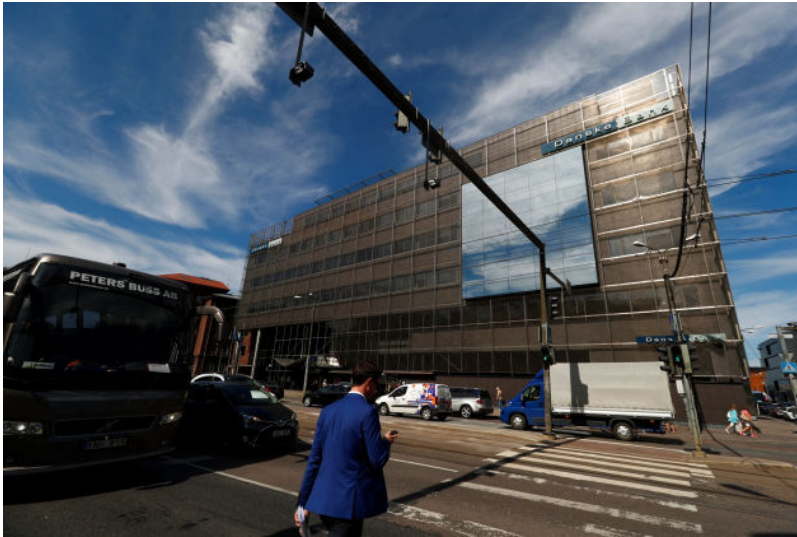
Danske Bank's Estonia office, a building once used by the Nazi military to produce radios and by the Soviets for tank parts.
